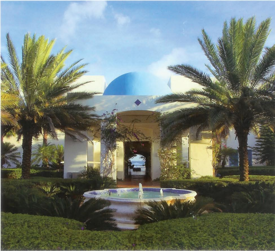
An elegant porte cochere entry welcomes guests to the CuisinArt Resort & Spa on the island of Anguilla. Looking through to the lobby, glimpses can be caught of the reflecting pool connecting to the powder-white sandy beach at the edge of the Caribbean. Cabinetics of Lakewood, NJ, provided cabinetry for the resort.
